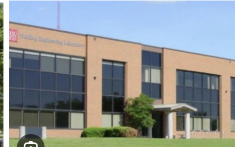
Edison Joining and Technology Center
