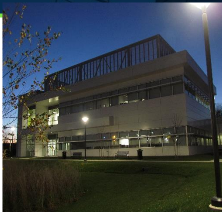
The Penn State Data Center houses CyberLAMP
